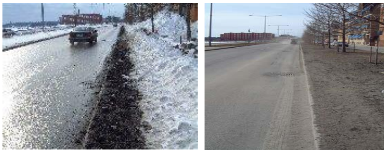
Figure 4 Pictures of the road side at Södra Hamnleden in Luleå, Sweden. At the Left, street during snowmelt and the right, street sediment left on road after final snowmelt (Westerlund, 2007).
