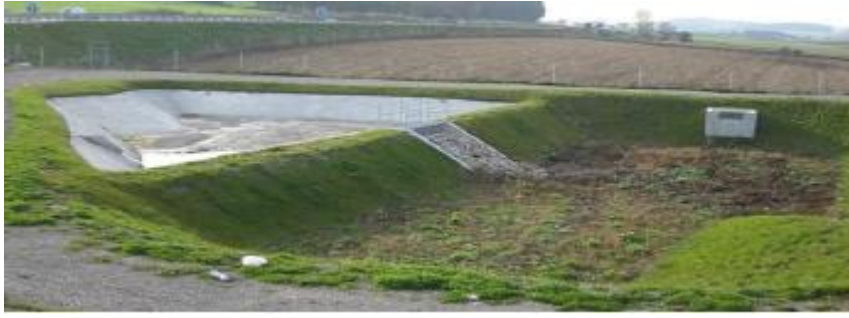
Figure 28 Standard system combining sedimentation and infiltration (photo: ASFINAG)
