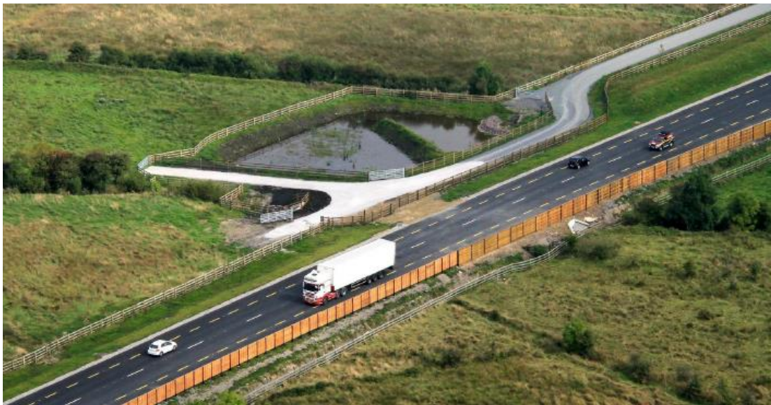
Figure 27 Example of SUDS in Ireland. Combined wetland, sedimentation, and attenuation facilities (photo: Transport Infrastructure Ireland)
