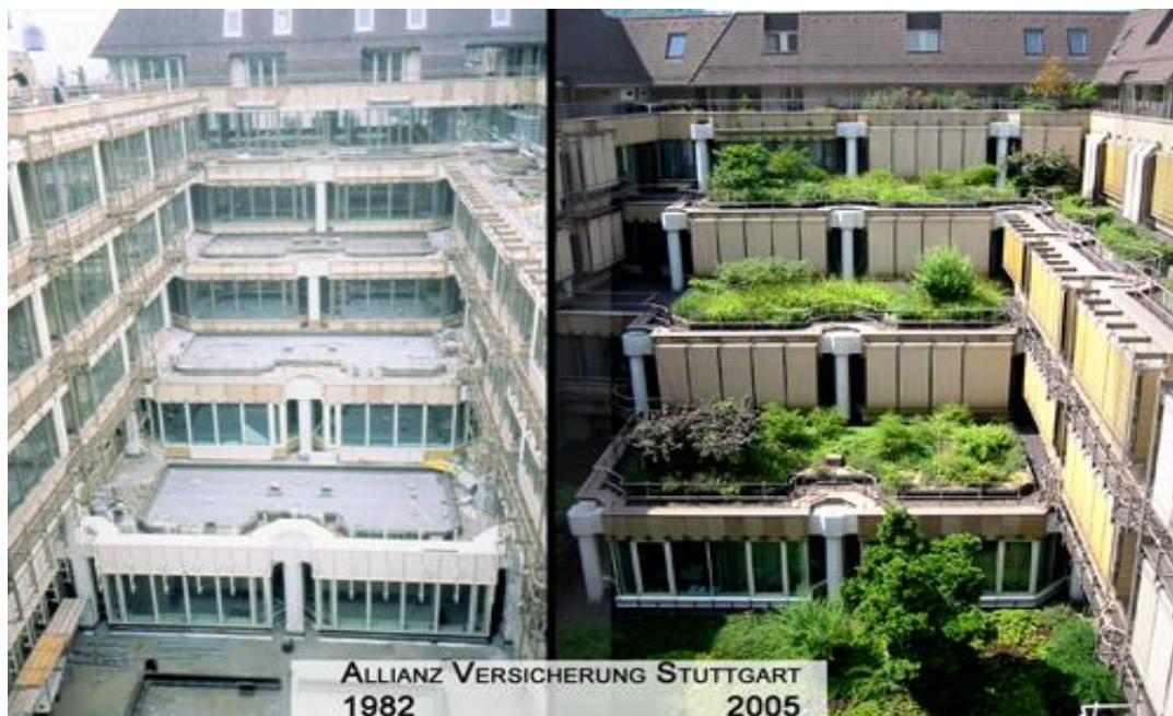
Figure 17 German company before and after green roof installation photo
