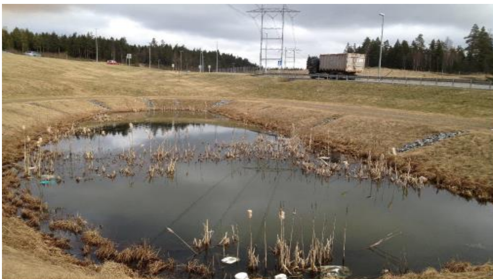
Figure 31 Example of a Norwegian sedimentation pond with a smaller pre-sedimentation pond (forebay, which can be seen in front of the band of vegetation crossing the pond) and a main pond (photo: Sondre Meland)
