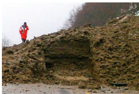
Figure 5: The vertical cut in the flank of this deposit shows that the masses consists of wet snow. (Frækaland, SVV)
