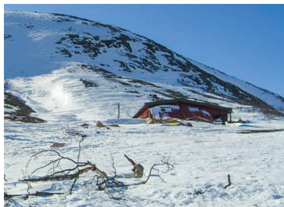
Figure 1: A slab avalanche has demolished a hut below a low hillside. (K Brattlien, NGI)
