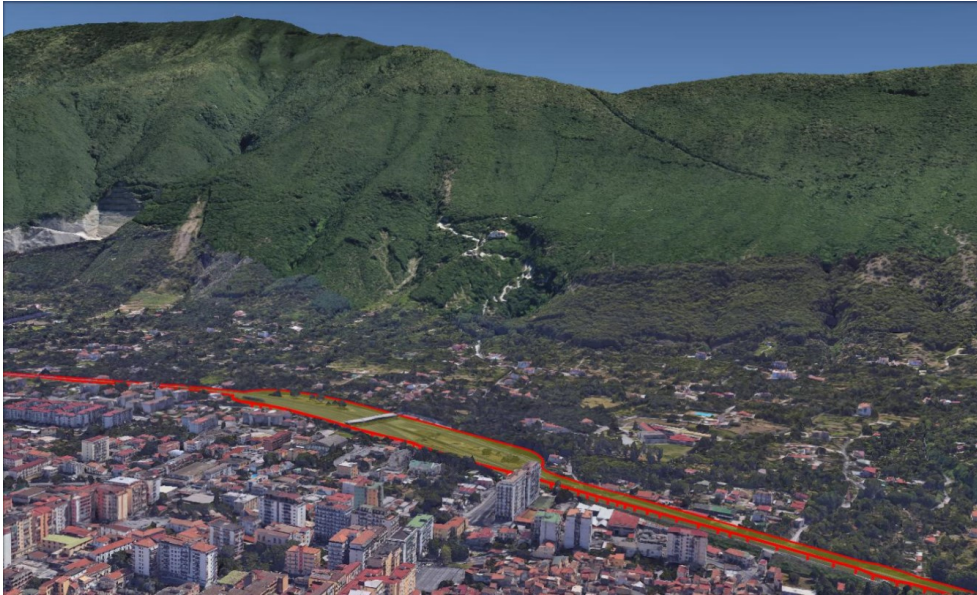
Figure 3. Infrastructure-scale view of the study area with the A3 Salerno–Reggio-Calabria motorway (boundaries marked in red).
