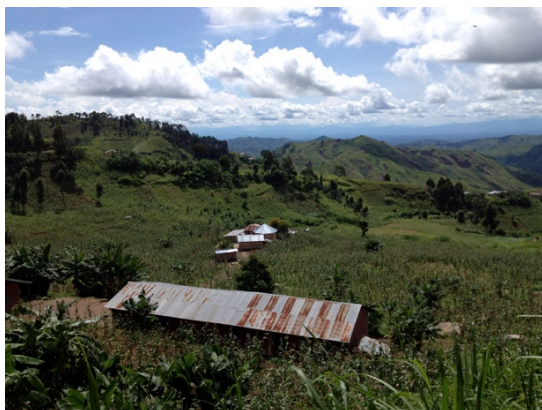
Figure 7. Kibuko primary school: Classroom building with farmland and storage house and teachers' house in the background. Photograph taken May 2014, Photographer: L. S. Jaeckle
