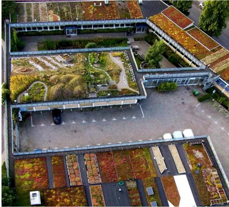
Figur 2.21: Augustenborg botaniske takhage (Scandinavian Green Roof Institute)
