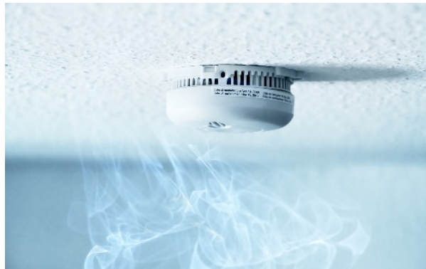
Figure 2 Smoke detector (NDLA, 2017)
