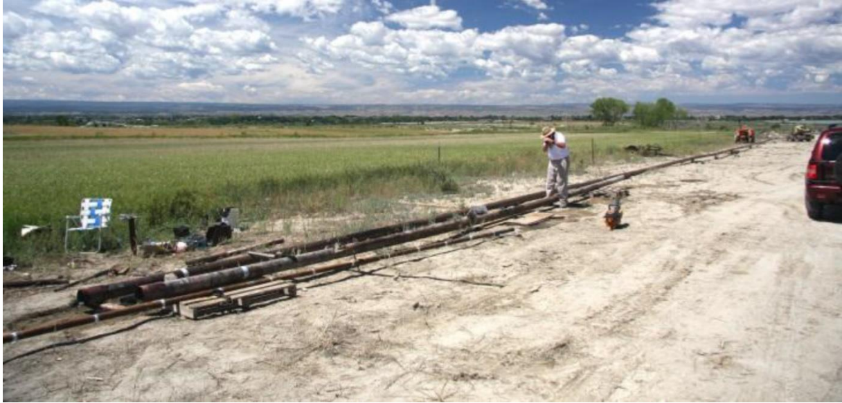
Fig. 15. The setup for the first full-scale compaction experiment (Oilfield Innovations 2013).
