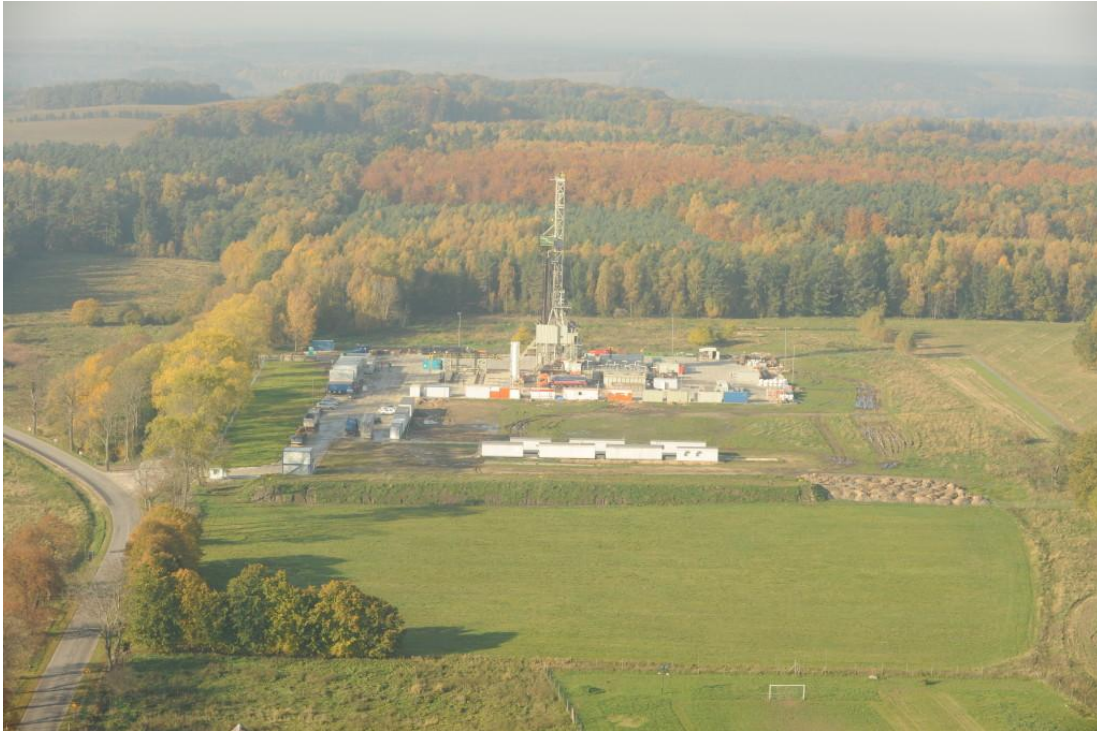
Figure 3 Wellsite in Strzeszewo (3legs Resources, 2015a)
