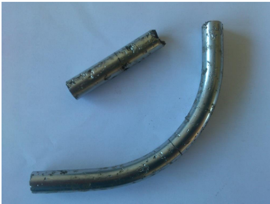
Figure 27: Corrosion on the body of Duplex after exposure at 60 \text{ }^\circ\text{C}
