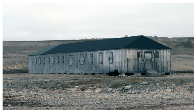
The main building at the Kinnvika station had room for 15 people. Photo: S. Elvevold.
