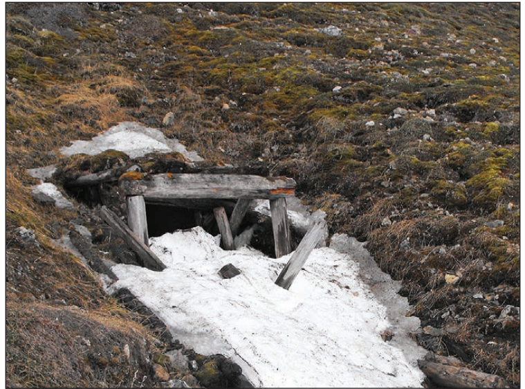
Figure 32 Gelifluction steps to the side and above mine entrance. Note how rock fall is caught on the surface of each step (Sessford, June 2012)
