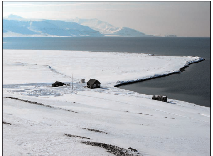
Figure 17 Buildings at Fredheim from left to right: Nødhytta (emergency hut), Outhouse, Villa, Gammelhytta (Old hut) (Sessford, May 2012)
