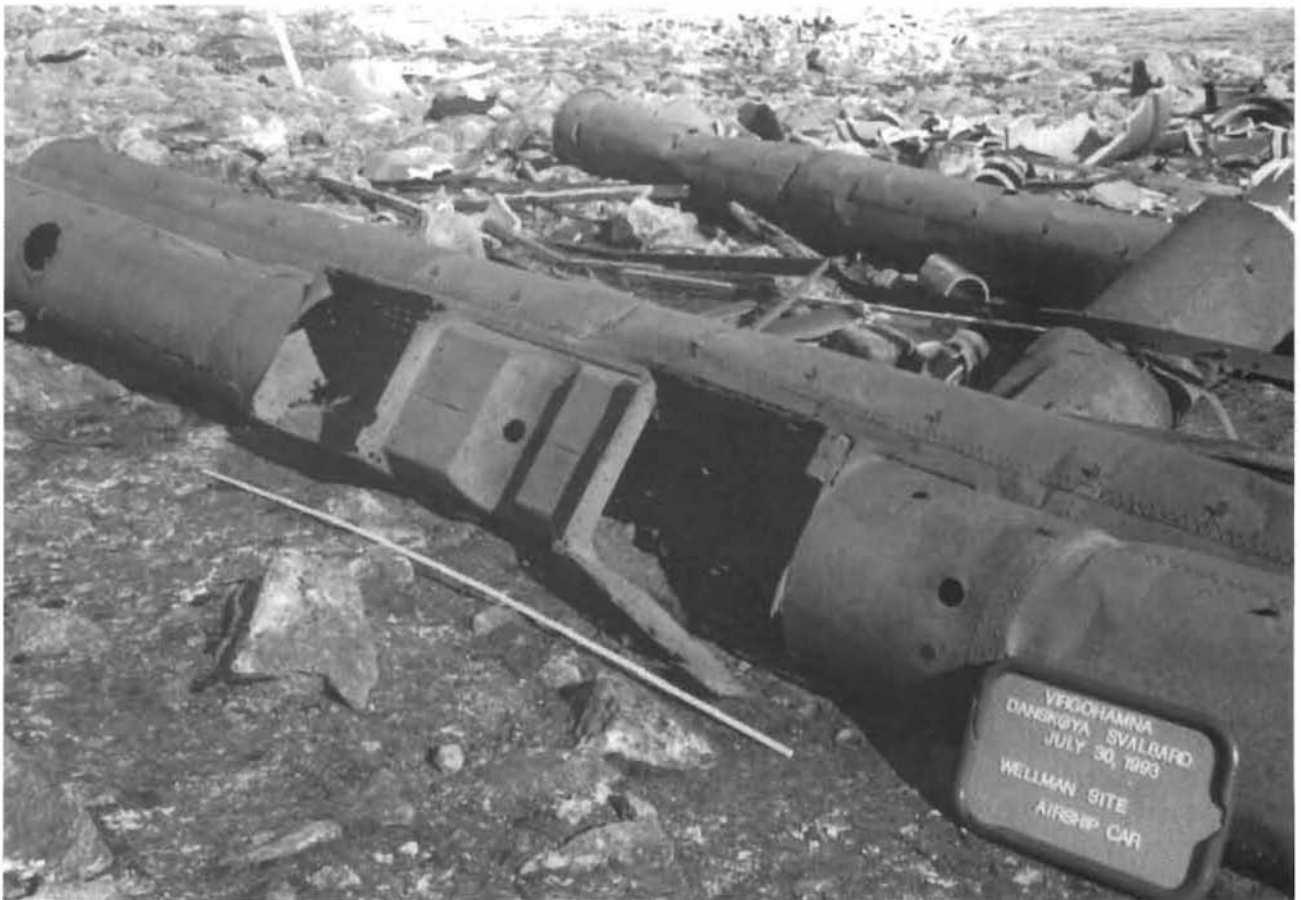
Fig. 50. Detail of the 1907–1909 airship fuel tank showing where engines were attached, 1993.
