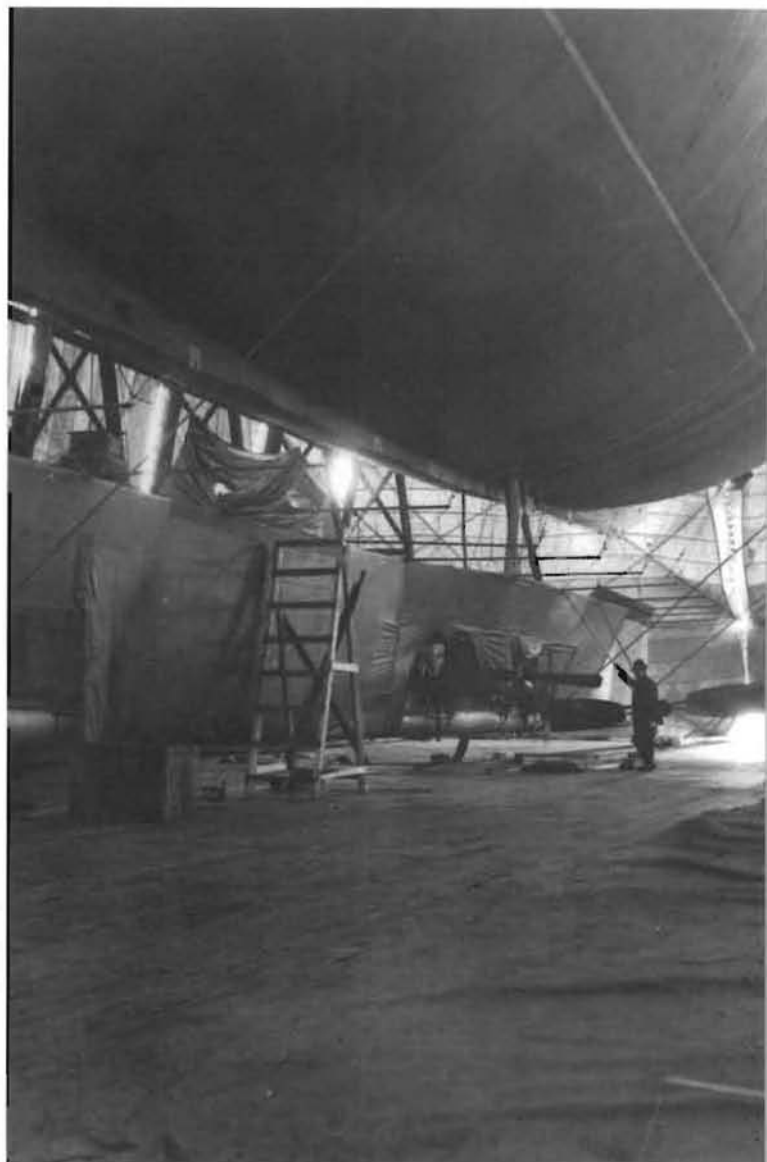
Fig. 8. Vaniman’s redesigned nacelle attached to the gas bag inside the hangar at Virgohamna, 1909. Photograph courtesy of Norsk Polarinstitt.
