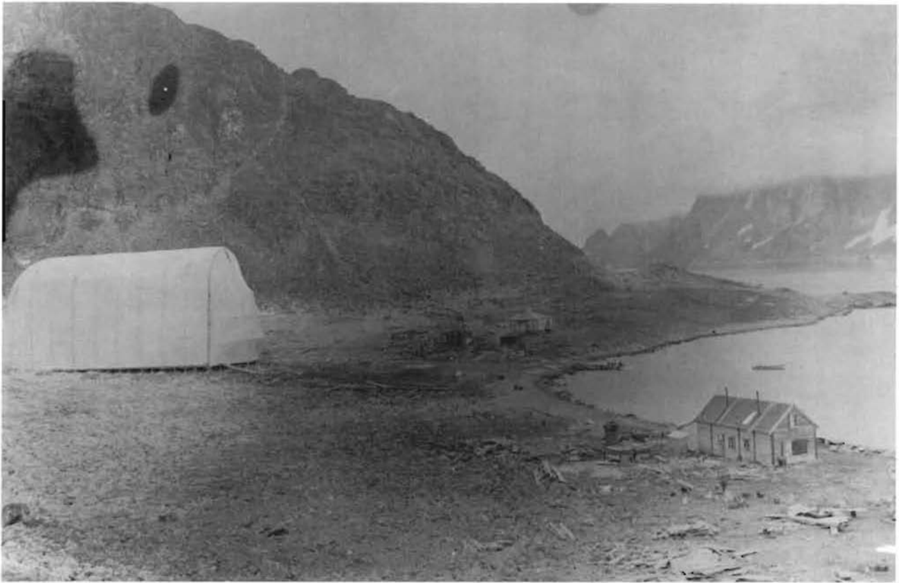
Fig. 6. View of Camp Wellman showing the airship hangar covered in sailcloth. Wellman's house and the ramp leading from the hangar upon which the airship would be rolled out can be seen in center. Pike's house and the ruins of Andrée's hangar can be seen at lower right. Photo courtesy of Norsk Polarinstitut.
