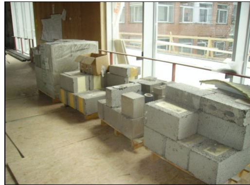
Figure 21: Allocated place for bricks inside the building
