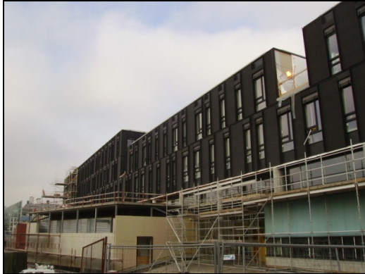
Figure 13: IFI2 under construction
