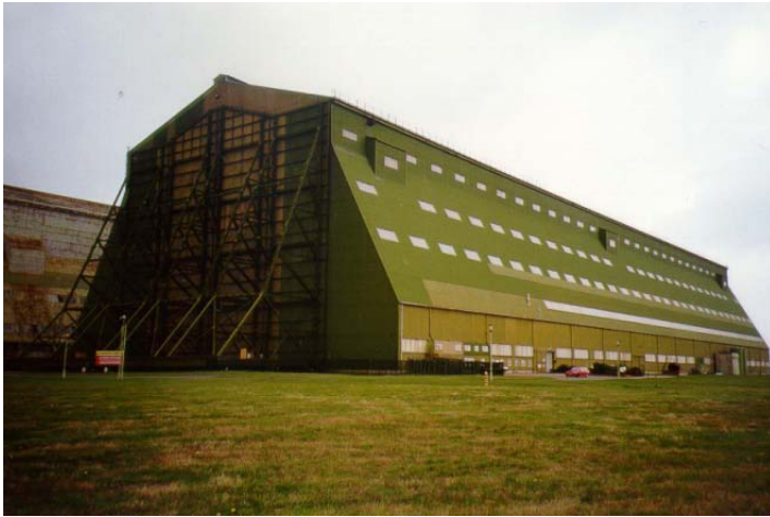
Figure 3.1. The old Zeppelin hangar near Bedford, UK.
