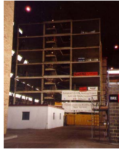
Figure 3.2. The Cardington Building
