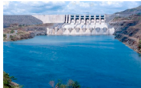
Picture 1. Magat Hydroelectric Generation
