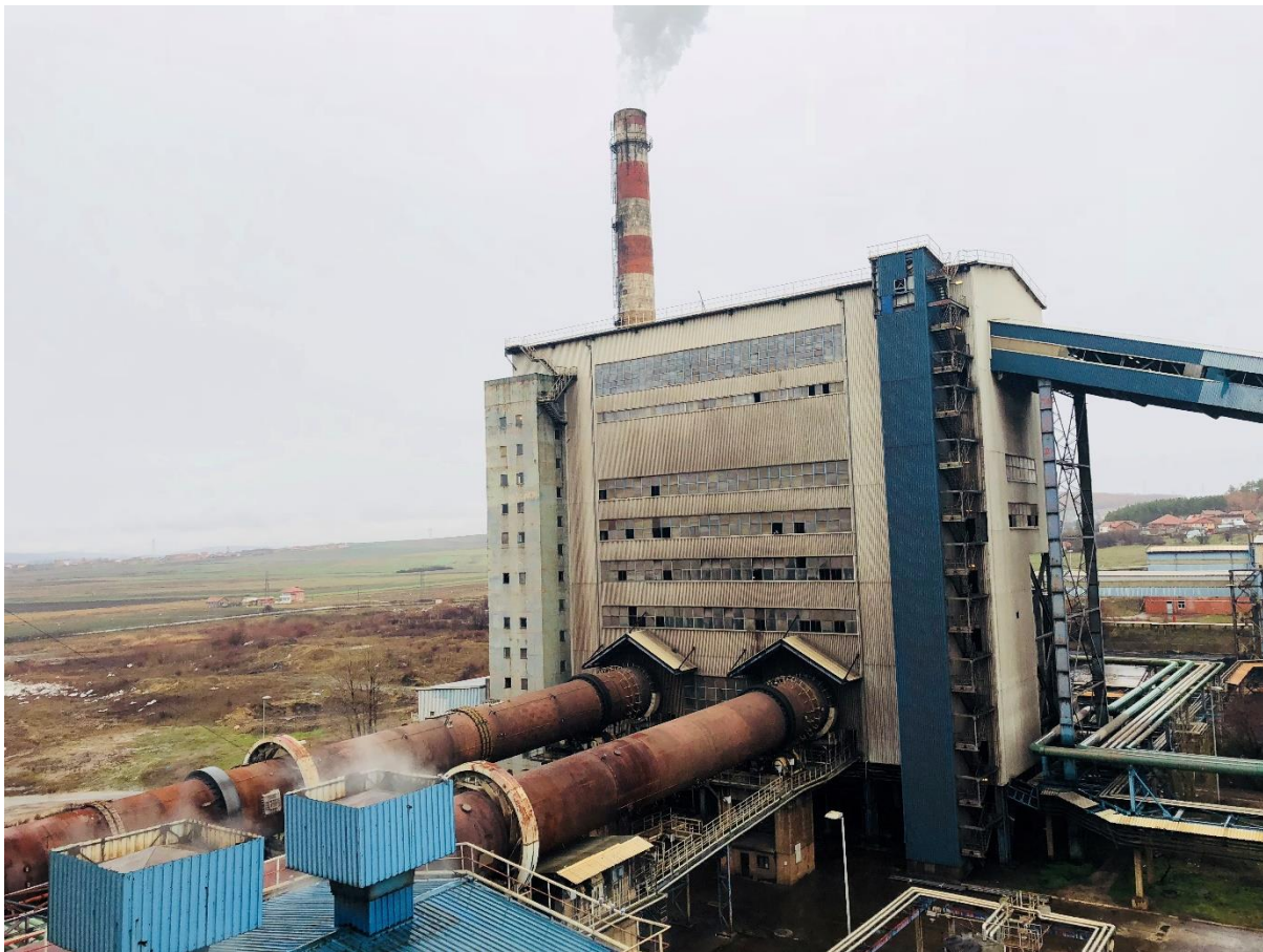
Fig. 1. View of Two Rotary Kilns in New Ferronickel in Ferronickel Street, 13000, Drenas (Glogovac) Kosovo.
