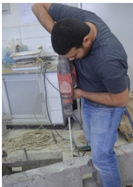
Figure 1: Drilling I.E. R technique
