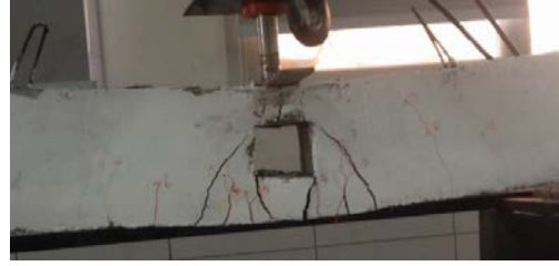
Figure 14: Crack pattern for beam F-R
