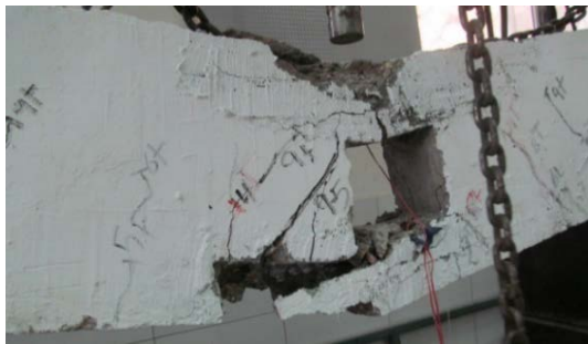
Figure 18: Crack pattern for beam F-R-N
