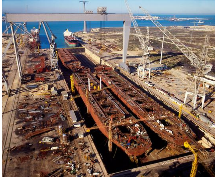
Figure 3-1 Graving dock with three newly built tankers in Cádiz, Spain (Mira 2014)
