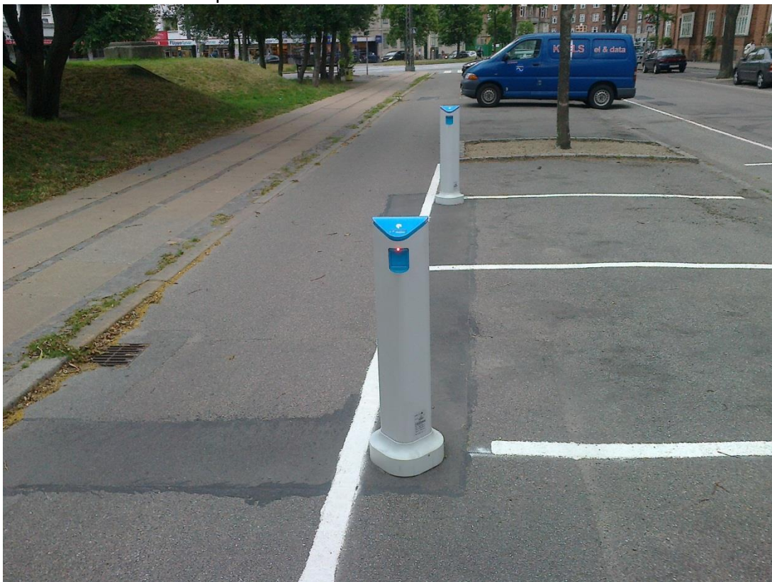
Figure 9: Better Place charging posts in Copenhagen summer 2013, shortly after the bankruptcy. Note the red light signaling out of service and the absence of electric cars. Photo: Mads Borup
