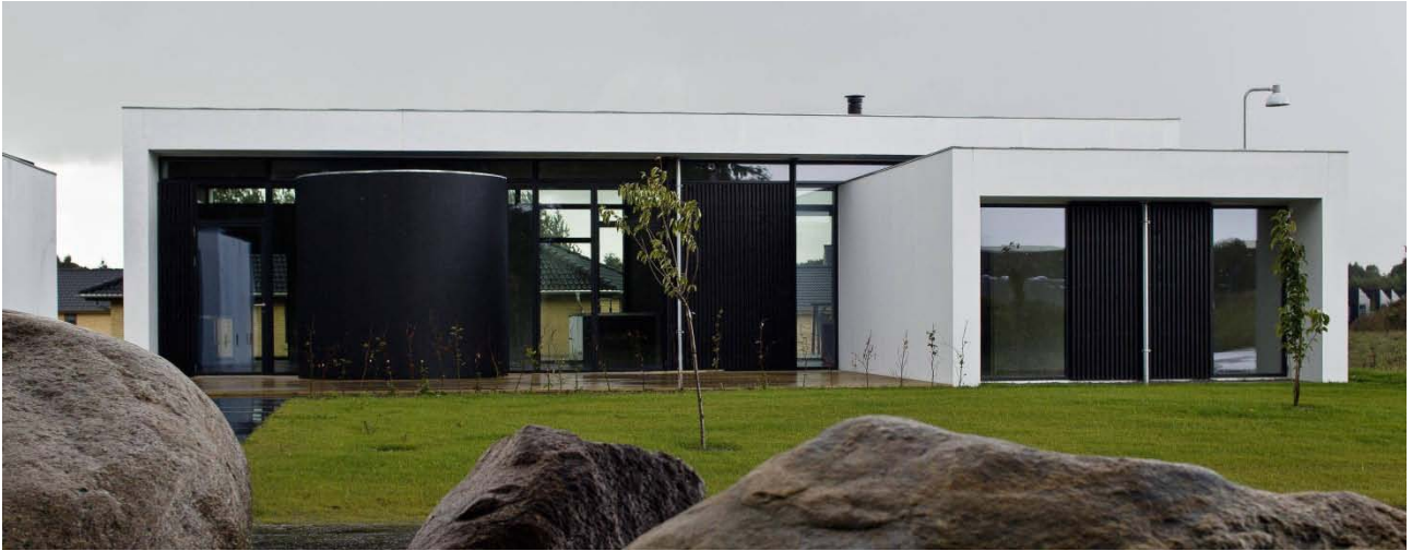
Figure 21: Villa Vid. A single family house made from HPC sandwich elements (connovate 2013 and Ingeniøren 2011)
