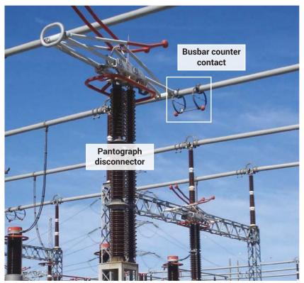
Figure 6. Pantograph disconnectors' busbar counter contact
