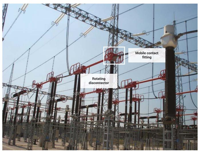
Figure 5. Rotating disconnector fitting
