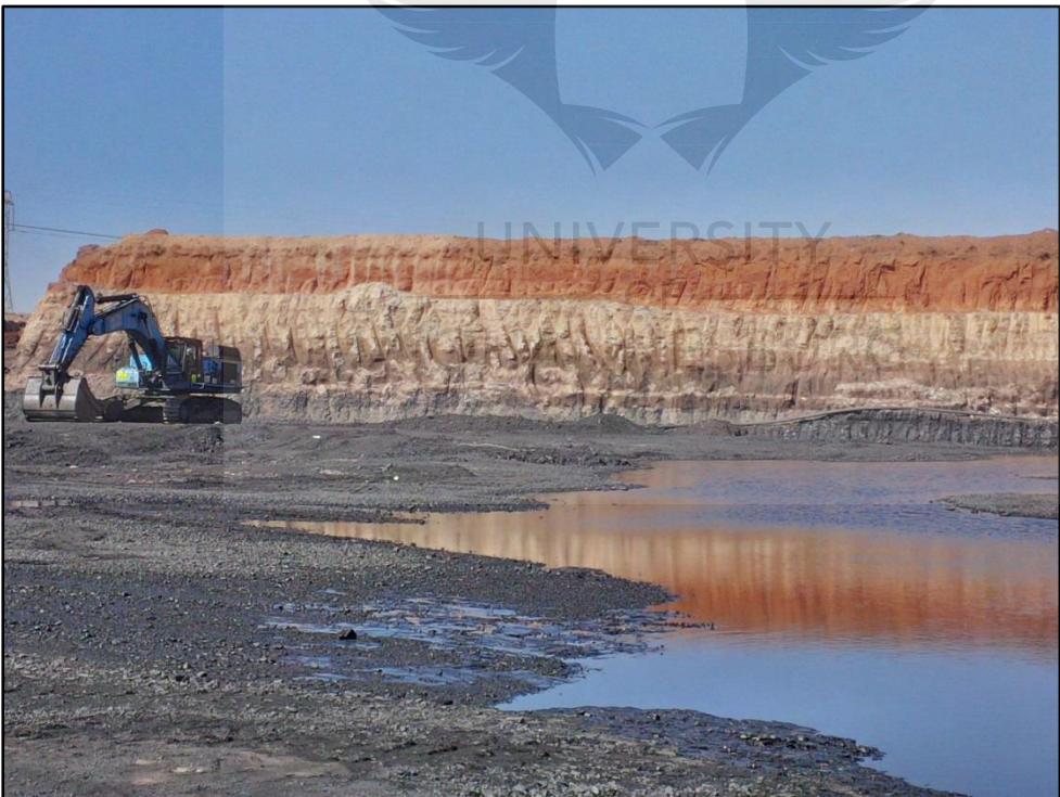
Figure 16: Pegasus South Pit during mining. Seam floor for Inyanda Seam 1 can be observed
