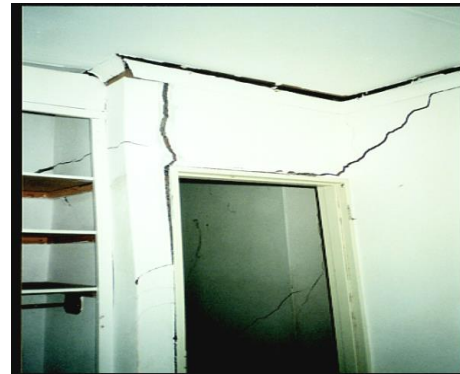
Figure 2: Superstructure failure
