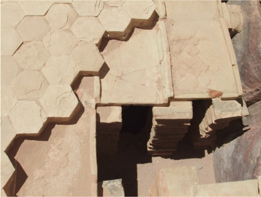
Figure 9. In situ roof tiles used in the floor construction of the winter triclinium (Room 14) with a hypocaust. Photo: Pirjo Hamari 2011.
