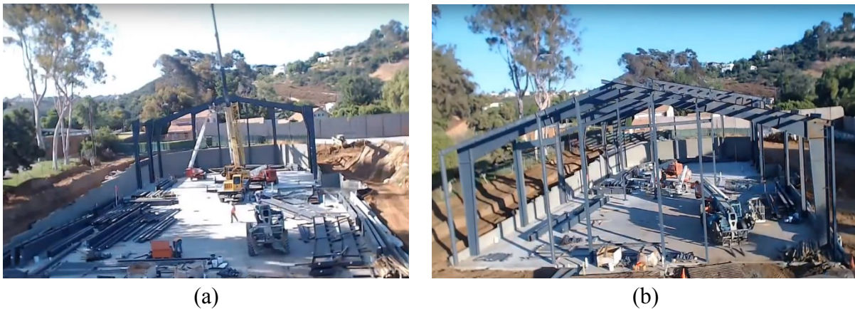
Figure 4-11 Snapshots of the construction of steel framed church (2019)
