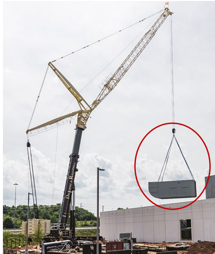
(a) In practice (Digging & Rigging, Inc., 2019)
