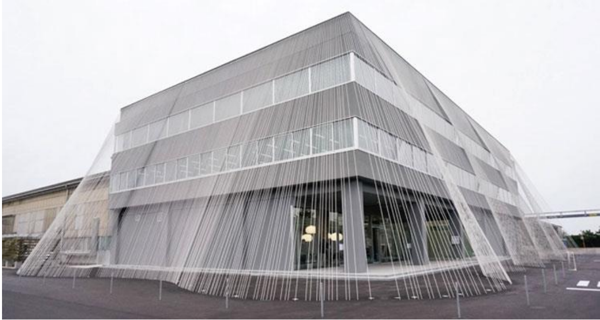
Figure 4.1-2: Komatsu Seiten's Head Office with CABKOMA Strand Rods. Reprinted from 'CABKOMA' by Komatsu Matere
