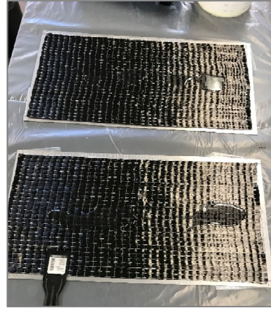
(b) placement of CFRP
