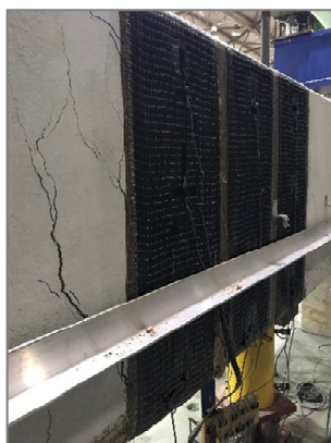
e) Shear and flexural cracks at the face of the column after test completion, and ruptured CFRP shown (east face)
