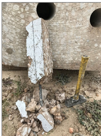
(b) concrete encased rebar after sledgehammer impact (stirrup)
