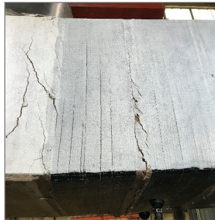
b) Major shear and flexural cracks after test completion (west face)
