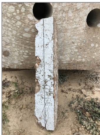
(a) extracted concrete encased rebar
