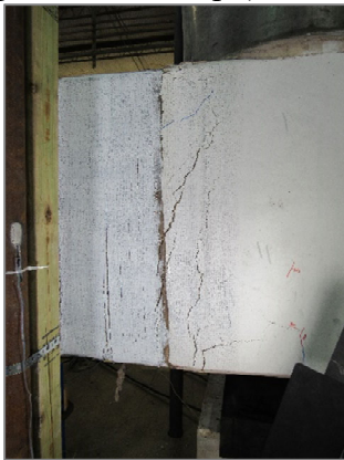
c) Major flexural cracks at the face of the column after reloading (west face)
