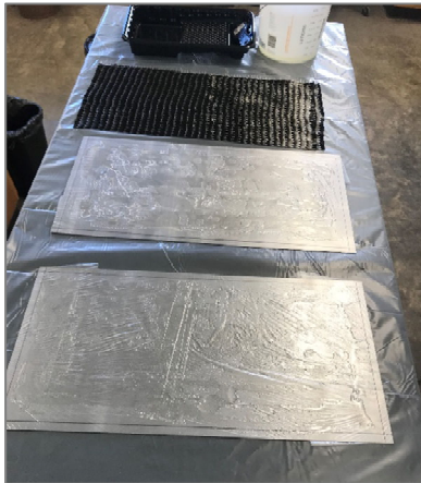
(a) epoxy applied to base plate surface
