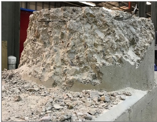
(a) Concrete cover removal
