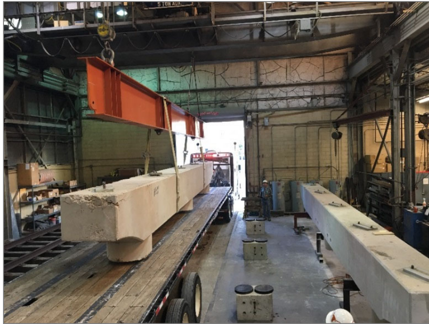
Figure 2.8. Receipt and unloading of Bent Cap 2 at FSEL (08/30/2017)
