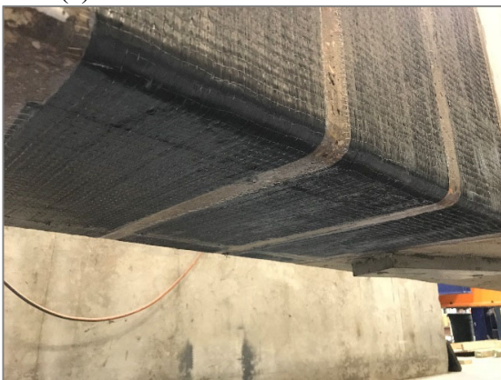
(c) bottom of finished retrofit
