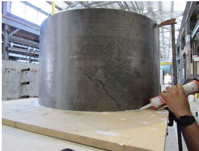
Figure D.8. Waterproofing of steel tube base and clamping of steel tube
