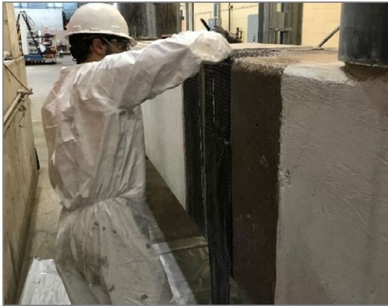
(a) CFRP strip application
