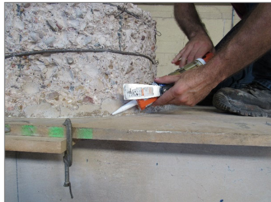
(b) caulk application to waterproof waterproof gaps
