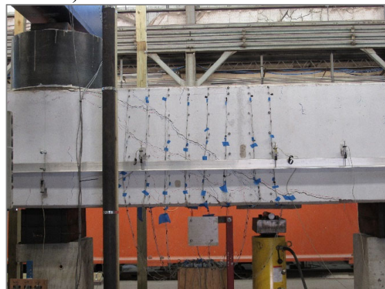
d) Major shear crack on the interior span after test completion (east face)
