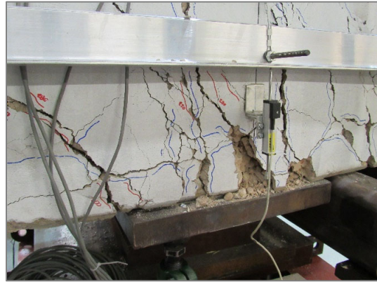
d) Concrete crushing at the added support bearing (west face) after cap failure
