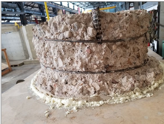
(a) foam application between MDF form and column stub outer face
