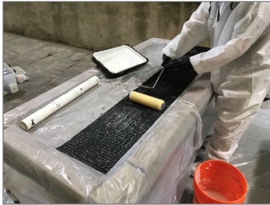
Figure D.11. Saturation of CFRP strip using a roller
