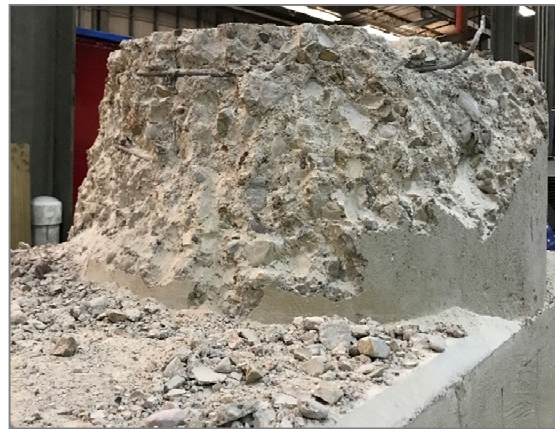
(b) concrete cover removal from BC1 south column stub
