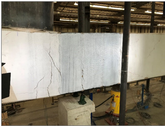
a) Major shear and flexural cracks after test completion (west face)
