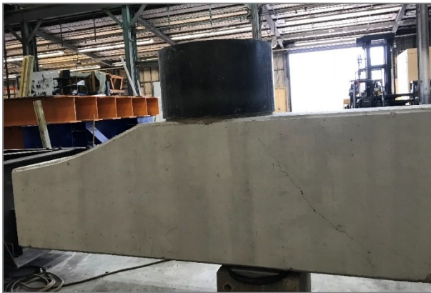
(b) Interior span 1 prior to retrofit
