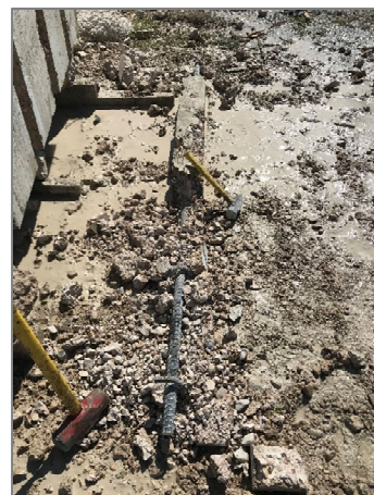
(c) concrete removal from longitudinal rebar
