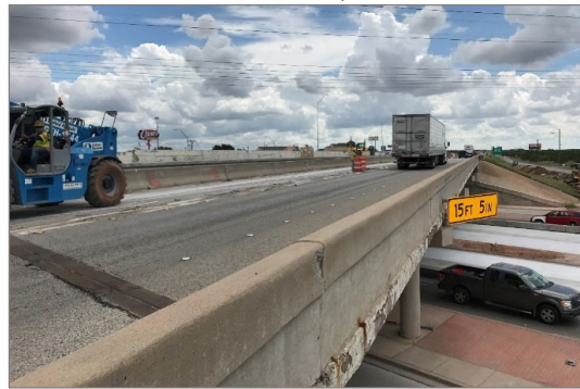
(h) bridge in service prior to removal
