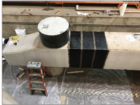
(b) overview of finished retrofit
