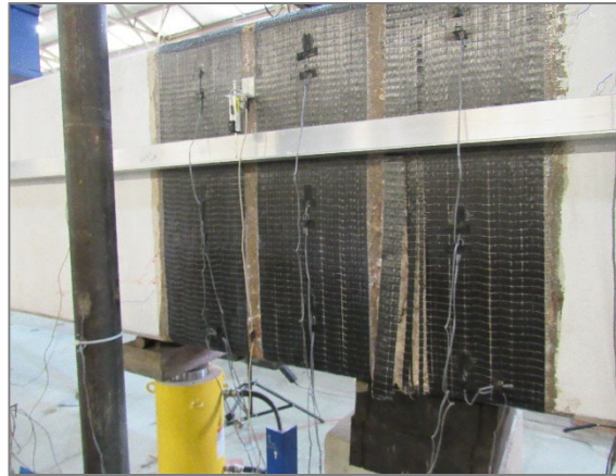
b) Delamination and rupture of CFRP at location of major flexural crack (east face)
