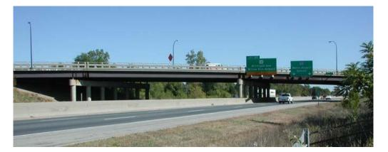
**Fig. 11.** Photograph of highway bridge in South-east Michigan where a SHCC link-slab was used in place of conventional expansion joint (Li, 2015)
