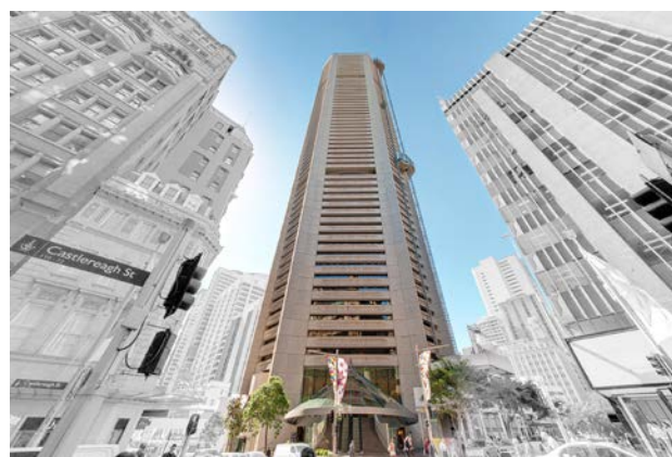
Fig. 1. Photo of MLC building
