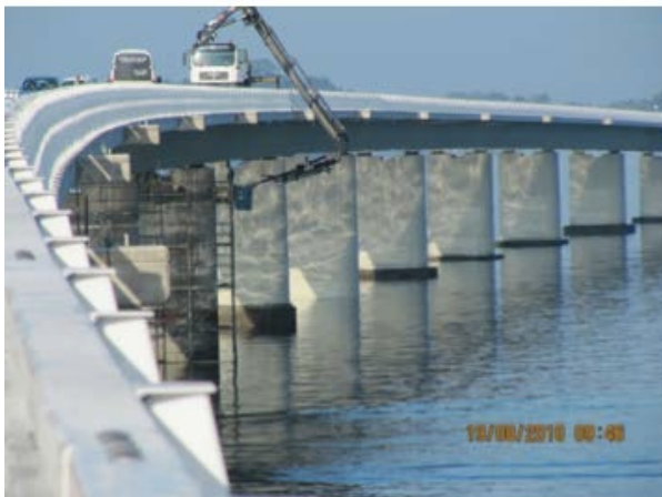
Fig. 7. Repair of the piles with the Fosroc jackets
