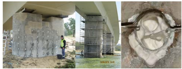
Fig. 8. Repair of the piles with conventional technique and CPT cathodic protection
