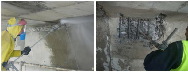
Fig. 4. Techniques of demolition of damaged areas of the deck.
