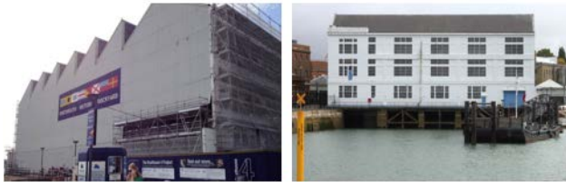
Fig.1. External side and rear views of Boathouse 4 structure
