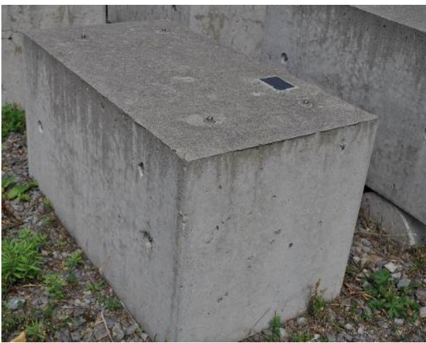
Fig.11. Condition of exposure block NMLiOH1.5 after 15 years outdoors (0.034% expansion)
