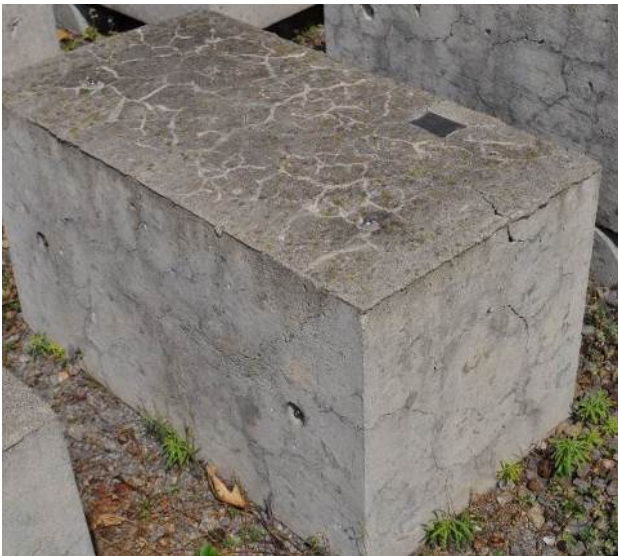
Fig. 9. Condition of control exposure block NM after 15 years outdoors (0.684% expansion)
