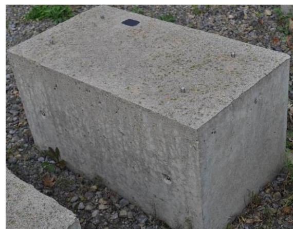
Fig. 19. Condition of block WyFA20LiN0.75++ after 15 years of storage outdoors (0.072% expansion)
