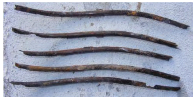
Fig. 1. Severe localized corrosion on prestressed wires extracted from about 40-year old Bridge in New Zealand (NZTA report 502, 2003)
