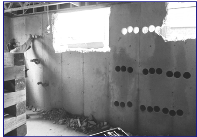
Fig. 4. Instrumentation for in-situ temperature and relative humidity measurements
