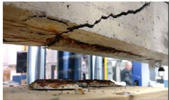
Fig. 9. Example of longitudinal cracking of severe corroded beam after load-bearing capacity test by three-point bending: weldable hot-rolled ribbed steel bar (A12-17), failure by shear
