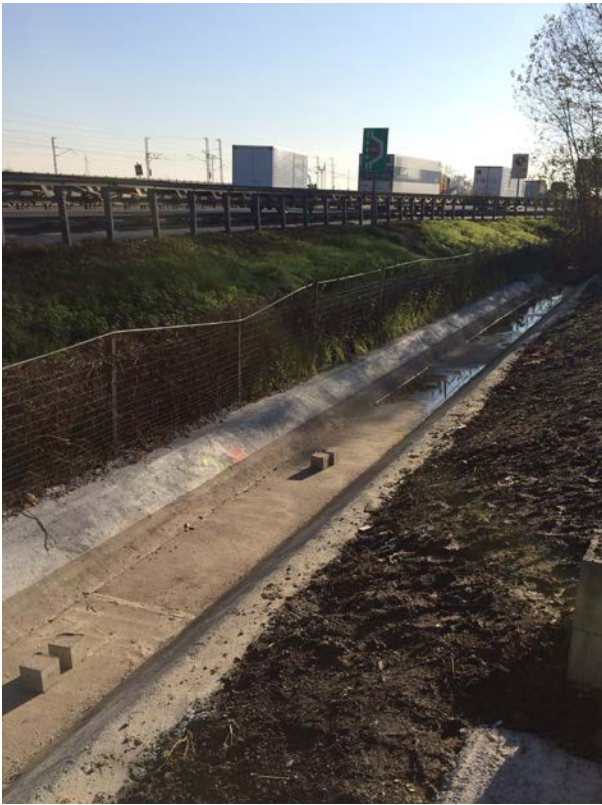
Fig. 3. View of the culvert
