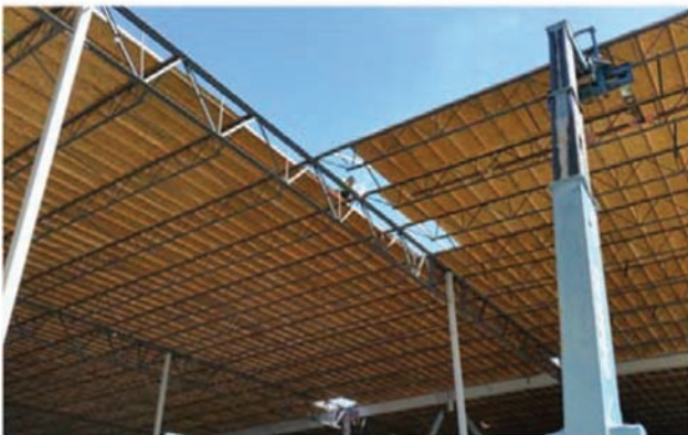
Figure 3.4 Panelized structure. (Source: http://www.dukepacific.com/projects/commercial-warehouse-panelized-roof )
