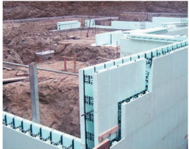
Figure 3.9 Insulated concrete form structure. (Source: https://decentralizedinc.com/the-anatomy-of-an-icf-wall/ )
