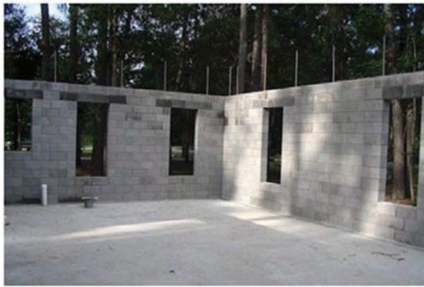
Figure 3.8 FlexLock block structure. (Source: https://www.seminarsonly.com/Civil_Engineering/mortarless-system.php )
