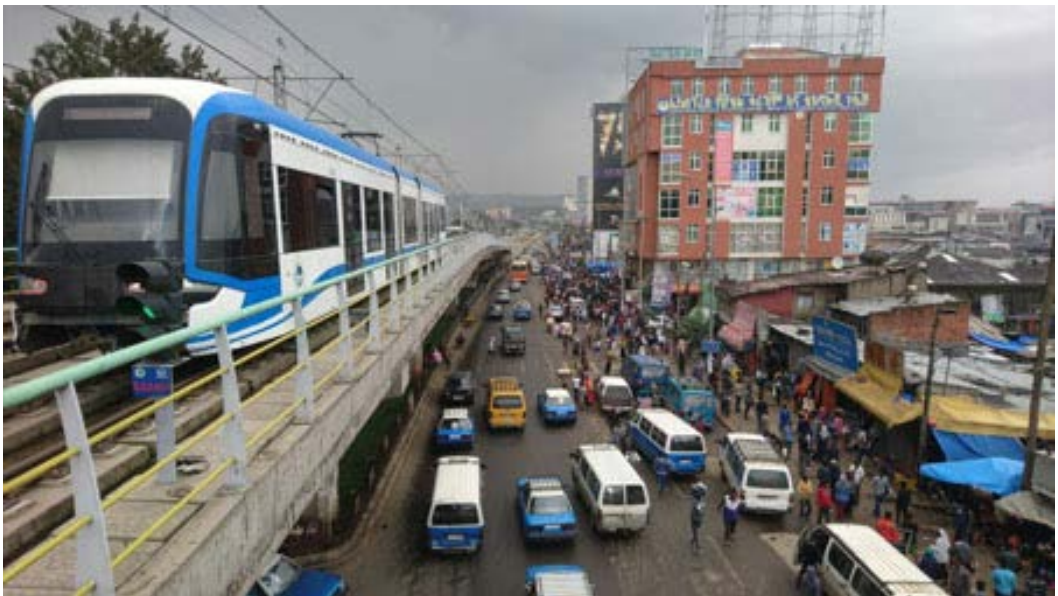
Figure 1. Addis Ababa’s Light Rail Transport System.
