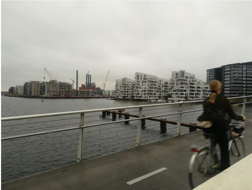
Figure 11 Brygge Bridge, Copenhagen
