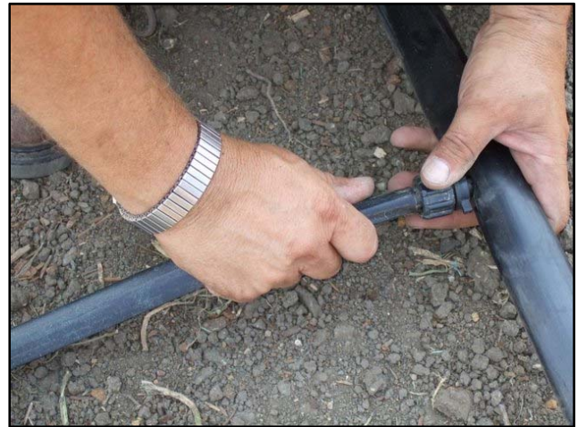
Figure 15. Connecting drip irrigation lines.
