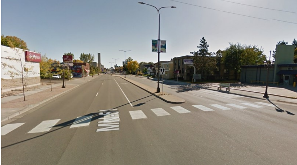
Figure 3.5 The crosswalk at Snelling & Blair, a five-lane road divided by raised median. Image taken from Google Maps.
