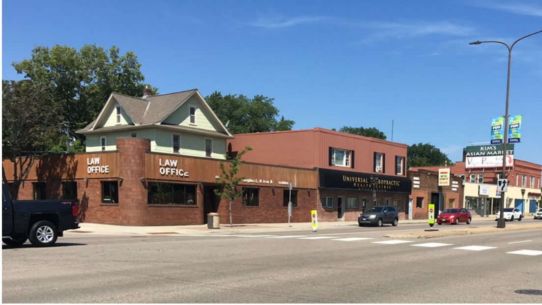
Figure 3.15 Snelling and Blair split gateway configuration, north side of crosswalk
