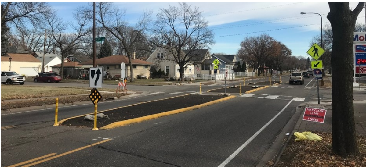
Figure 4.6 The crosswalk at Maryland and Duluth, a two-lane road separated by a pedestrian refuge/road diet.
