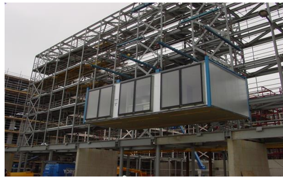
Figure 2: Light steel framework of a module Figure 3: High-rise modular building, Manchester, UK
