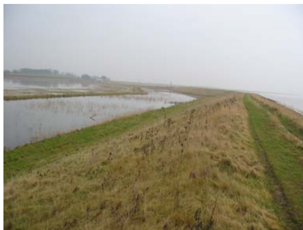
Figure 3.11: Photo of the landward face of the embankment (reprinted from [74])
