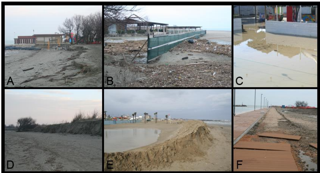
Figure 6.3. Impacts of the event in February 2015 on the Lido degli Estensi-Spina case study area. Impacts of erosion and flooding on concessions at Lido di Spina south (A, B) and Lido degli Estensi (C); sandy scarp due to the erosion of the dune in the south of Lido di Spina (D); eroded Winter Dune in Porto Garibaldi (E); damages to the Porto Canale front at the Lido degli Estensi (F).
