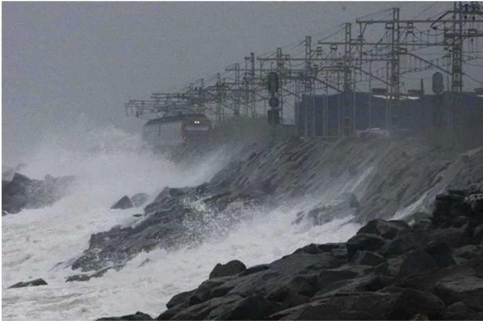
Figure 4.5. Affection of the coastal railway along the Maresme coast during the impact of a storm on March 2003.
