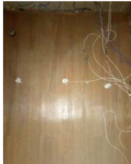
Figure 2.17 Finished radiant heating floor [14]
