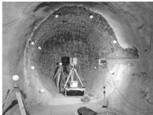
Figure 7. Laser scanning of excavation surface of tunnel (from [17])
