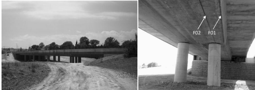
Figure 24. Viaduct Road BP-1413 in Cerdanyola del Vallès (Barcelona) (from [49])
