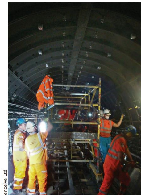
Figure 11. Wireless tilt meters installed on cast iron tunnel segments before grouting works (from [23])
