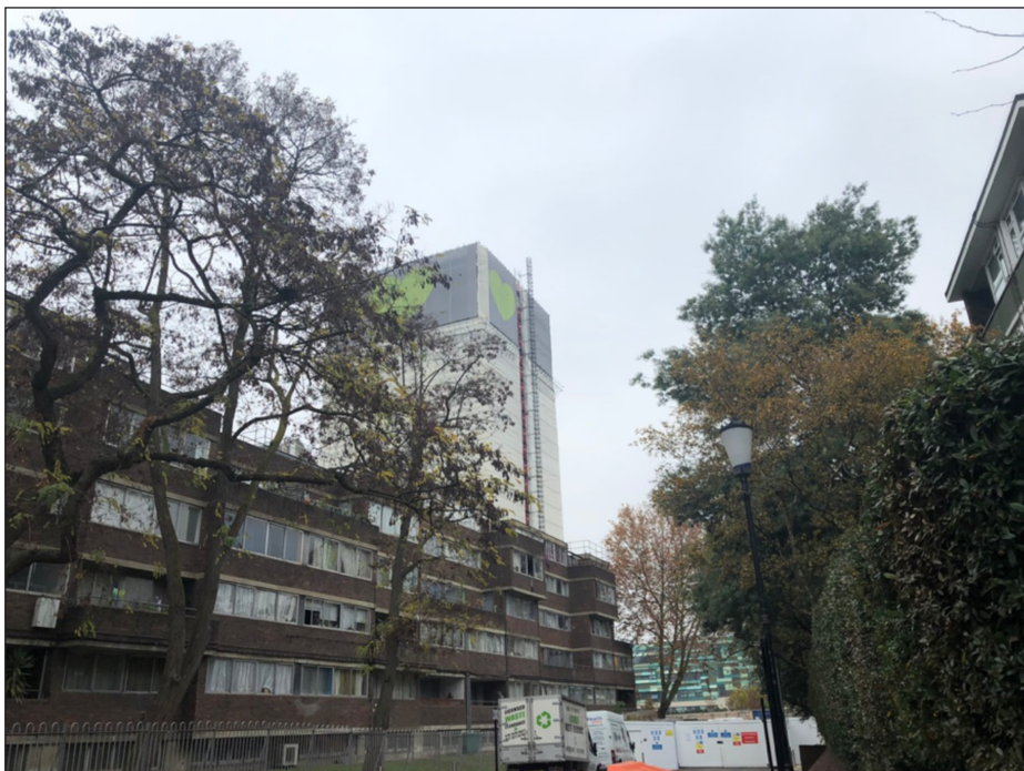
Figure 2: Grenfell Tower – identified by the Grenfell Green Heart – under reconstruction in the heart of high density housing area, Notting Dale, November 2018. (Photo credit: Samantha Owen).
