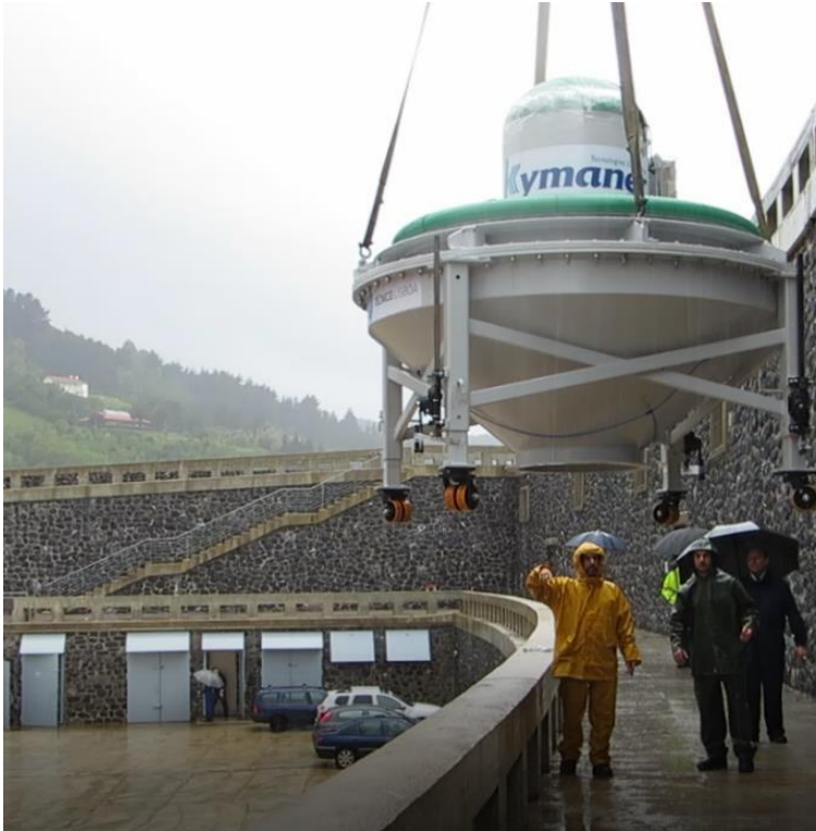
Figure 13 Kymaner turbine at Mutriku for testing
