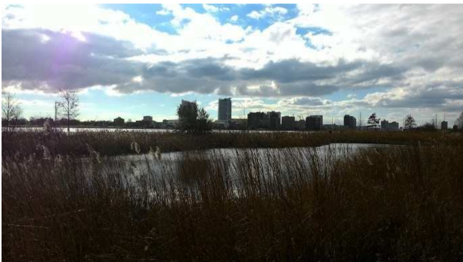
Fig. 1.4. Example of an artificial wetland for the depuration of urban stormwater (Detroit, Michigan, USA). Treated water is discharged directly in the Detroit river.
