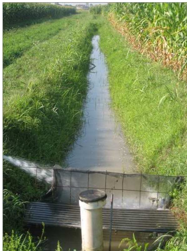
Fig. 2.4. Example of a delivery ditch during subirrigation. The modular riser in PVC prevents water to flow out of the ditch until the water level reaches the riser level. On the left, water is pumped into the ditch for subirrigation purposes.
