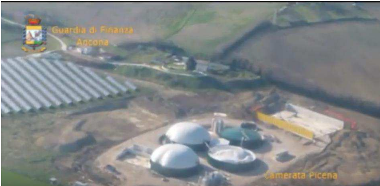
Helicopter view of a biogas plant under investigation close to PV systems on the ground. Source: Media material (2013)
